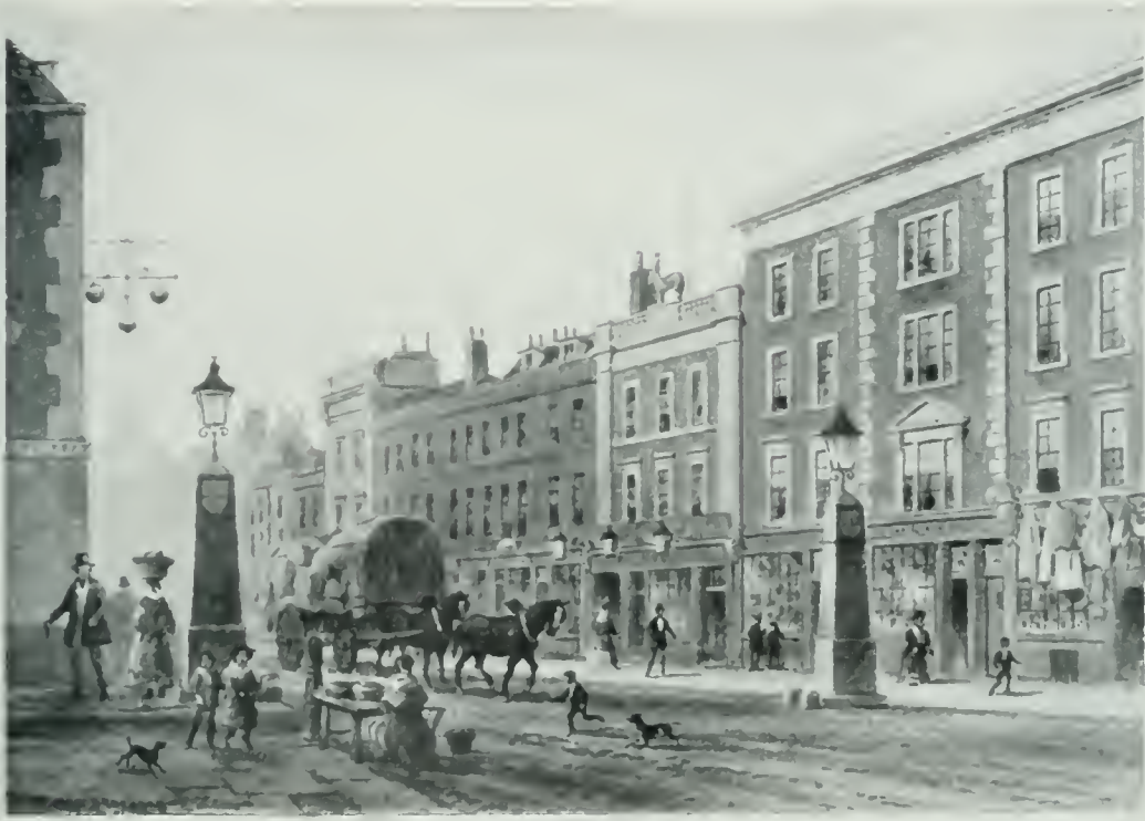
OLD VIEW OF THE CITY BOUNDARY, ALDERSGATE STREET ( b. 332).
